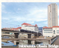
Takarazuka Onashi Bridge
